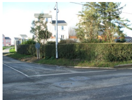
New Sheetlend Road footpath and improve- ment works complete
